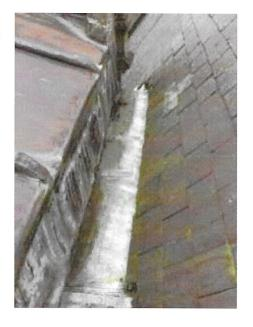
1.8 A number of slates have been damaged or come loose on the chancel at the junction with the gutter. Patching of the slates appears to have averted water penetration but several require refixing.
