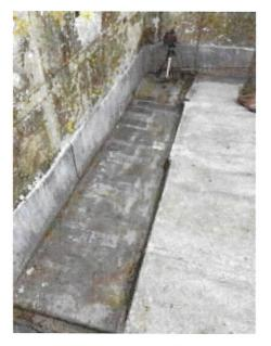
2.5 At the west end of the parapet gutter is a raised section that has a lead covering from a former flue outlet. The flue is now redundant and the liner/lead could be removed to below the roof line to improve/simplify the detailing in this corner..
