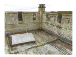
2.2 As with the organ chamber roof the leadwork to the tower roof has a number of splits that have been repaired and several sheets have slipped down the slope. Although the lead sheets are smaller than on the organ chamber they are still relatively large for their thickness and are of a reasonable age.
