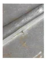
1.3 On the north slope the western bay lead has slipped down the roof slope.
