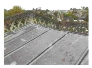
1.2 On the south slope there are numerous splits and patches to the leadwork. Several patches have split suggesting this is an ongoing problem. The bay sizes are too large for the code of lead which results in thermal movement within the lead causing the splits and damage. The patches are a mixture of welded lead repairs and bituminous patches.
