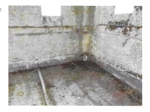
2.4 The lead parapet gutter to the north is in one long bay and has numerous splits and creases across the lead from thermal movement. The splits have been patched but due to the length of the lead bays it is likely that this problem will continue.
