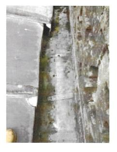
1.5 From the north gutter there is a lead chute outlet through the parapet wall. The lead has split and been patched with a modern coating.
