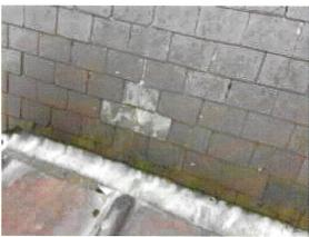
1.9 Flashings between the lead roof and parapets on the organ chamber roof have very poor upstands. The pierced decorative stone parapets severely restrict the available upstand. In several areas the pointing has failed and the flashings have become loose. The parapet gutter flashing has split in several places.
