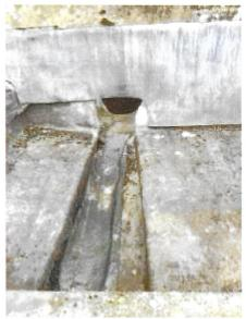
1.6 Between the eaves of the southern roof slope and the lead gutter on the chancel roof is vertical lead sheet cladding. Fixings to several of these lead sheets have failed causing the sheets to drop and sag.
